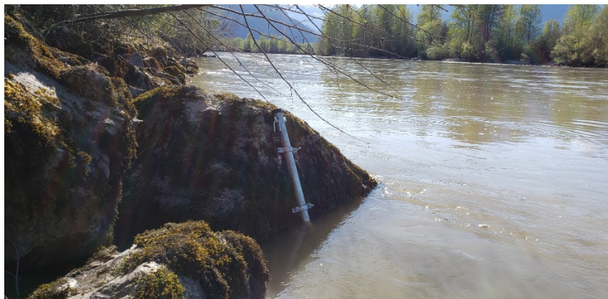
Photo 2.1 Levellogger stilling well fastened to rip rap boulder at DS Airport Bar station.
