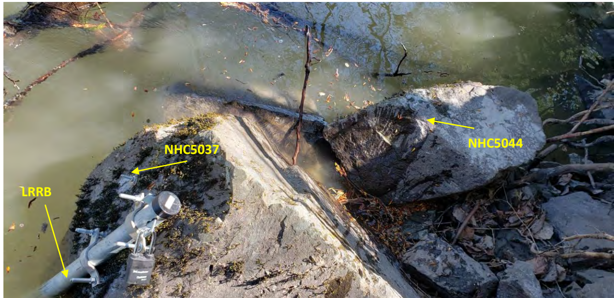
Photo 3 Rockbolt benchmarks NHC5044, NHC5037 and LRRB (lower right rock bolt) near PT pipe
