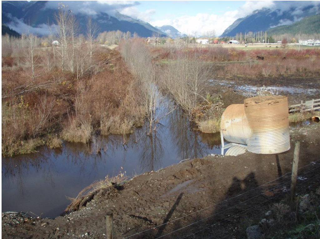
Photo 10 Arn Canal from the CN Rail embankment (upstream)
