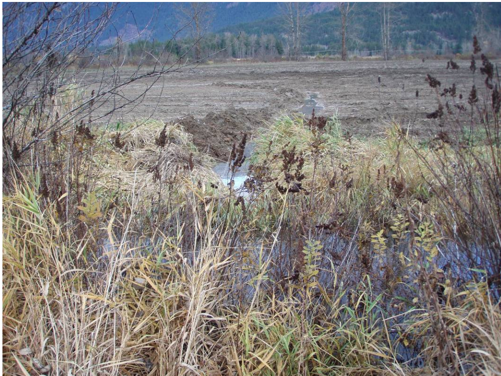
Photo 18 Arn Canal upstream of Collins Rd. – low freeboard (example 1)
