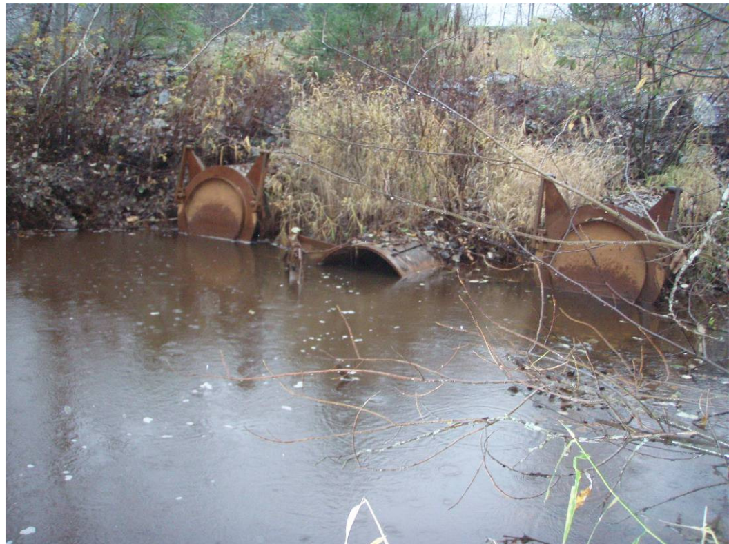
Photo 2 Arn Canal floodbox
