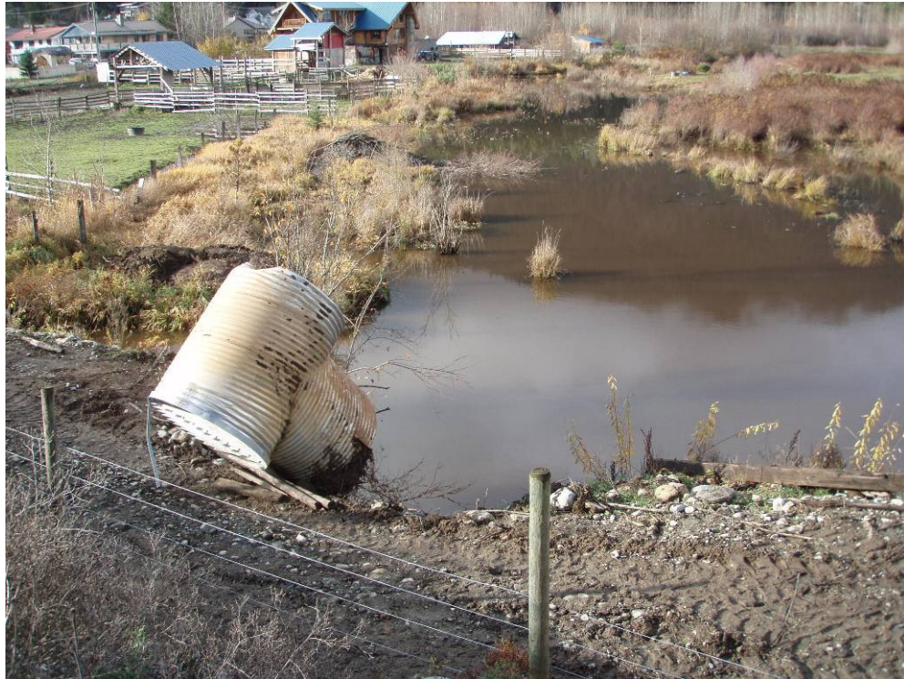
Photo 9 Wetland upstream of CN Rail embankment
