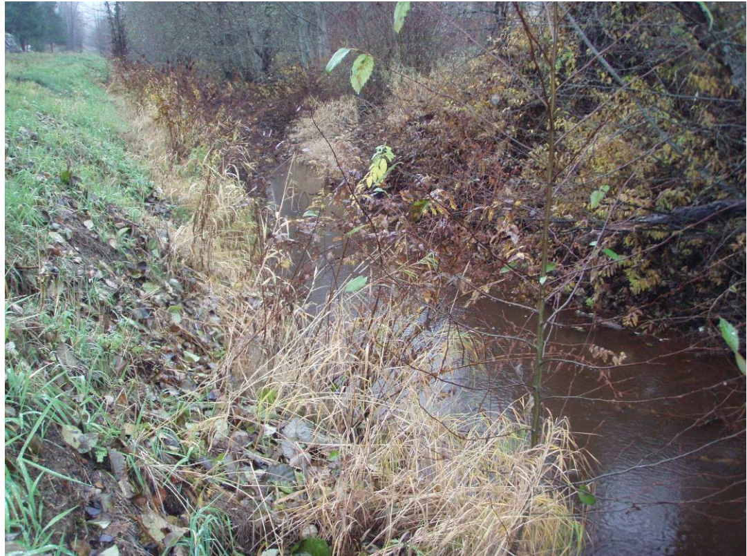
Photo 3 Arn Canal downstream of the Hwy 99 bridge
