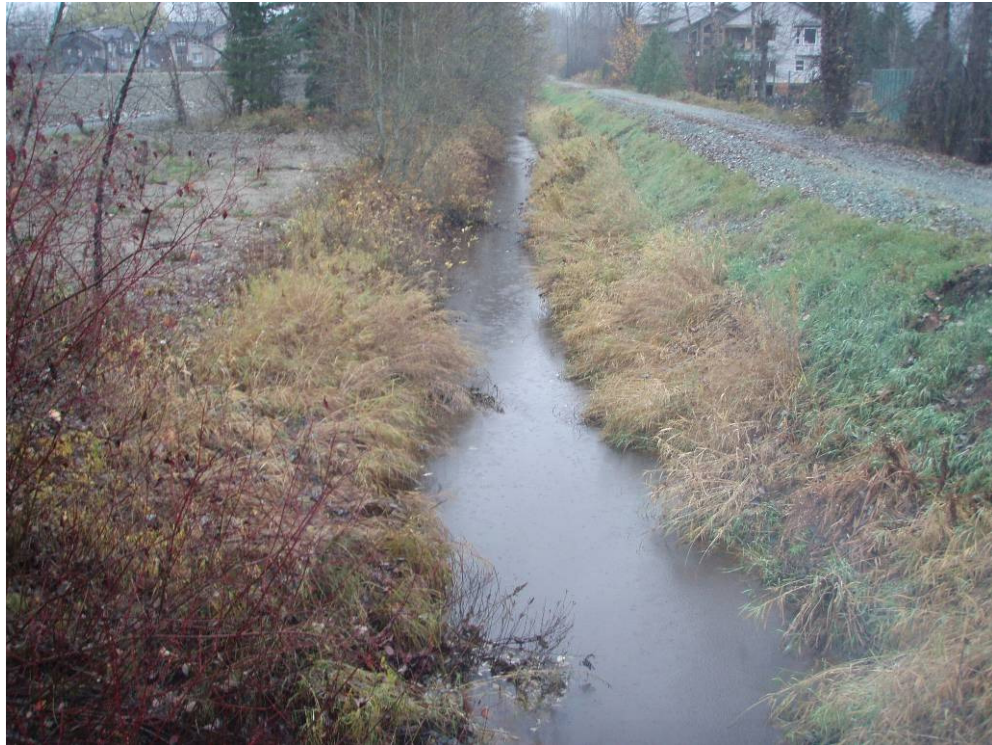
Photo 5 Arn Canal from the pedestrian bridge upstream of Hwy 99
