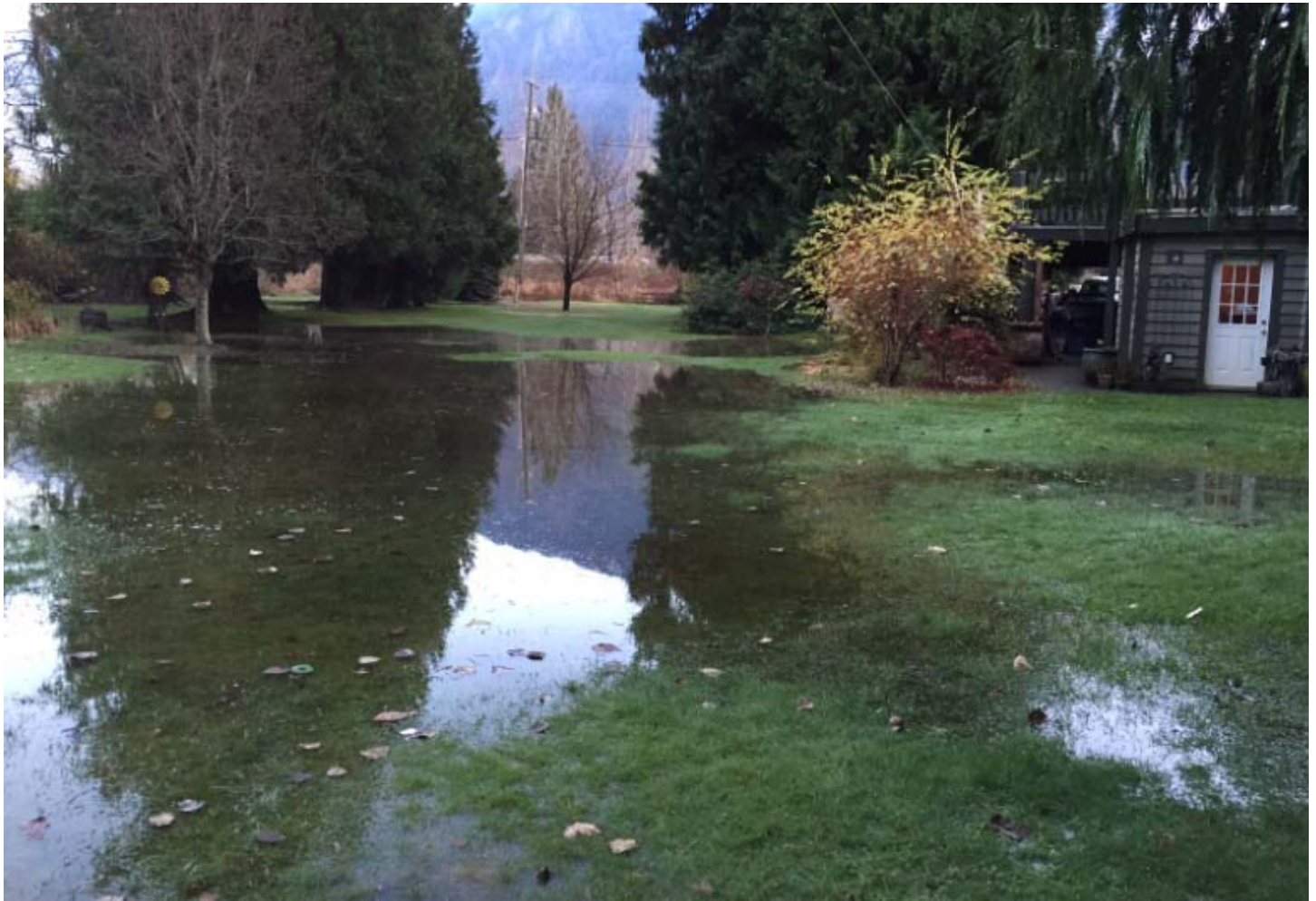
Miller Lillooet Dike Piping causing flooding on Oberson Property Nov 9 4:30pm.
