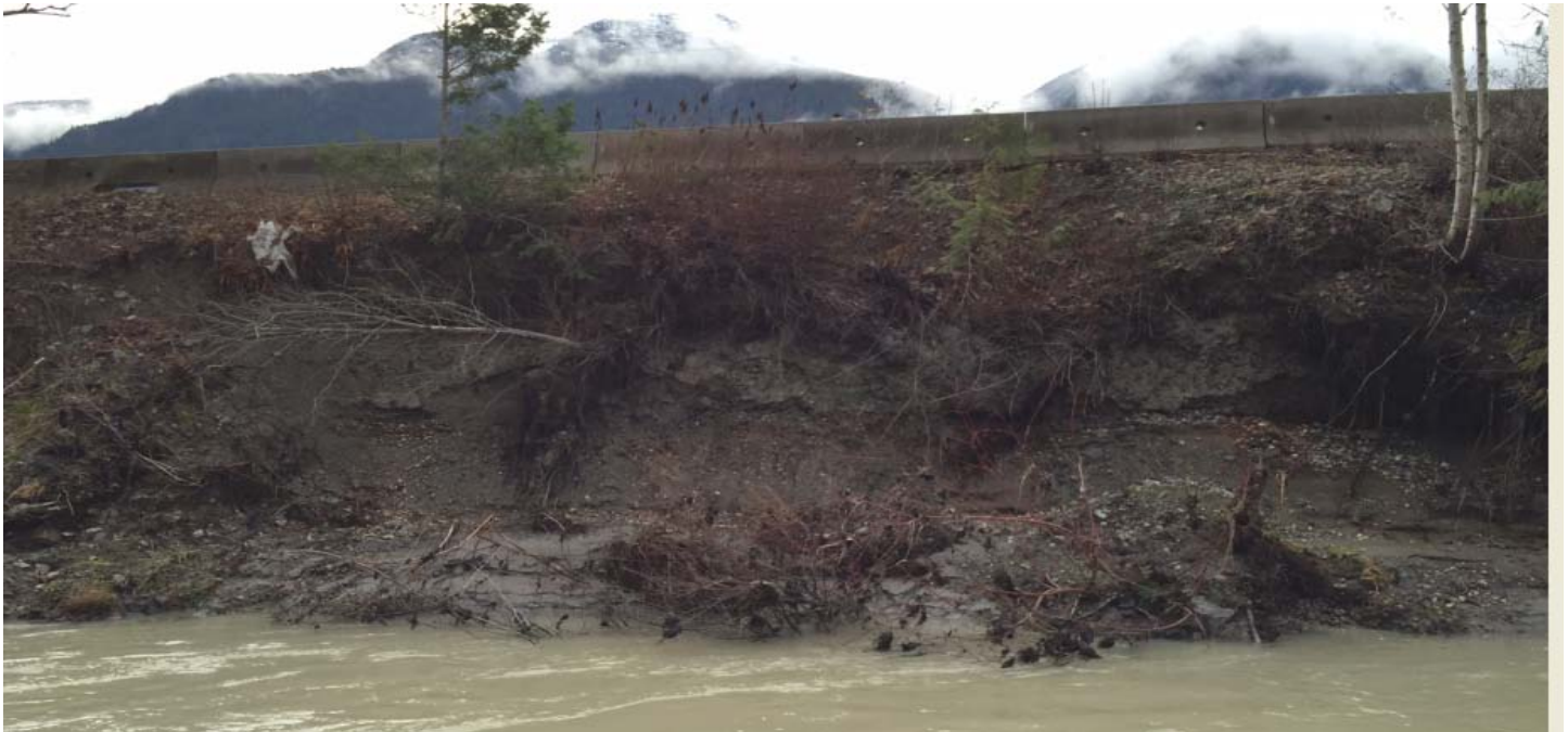
Meadows road Bank failure at Ronayne farm Nov 17 2016.
