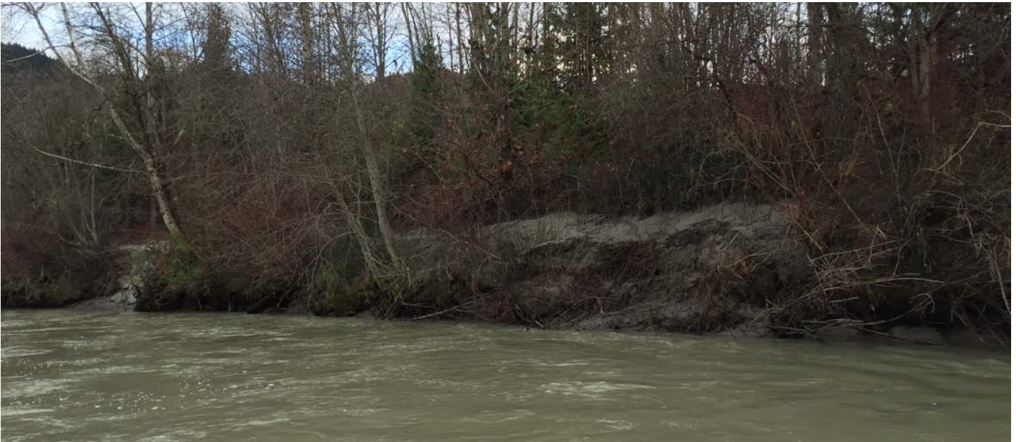
Ayers Dyke Bank Failure Nov 17 2016
