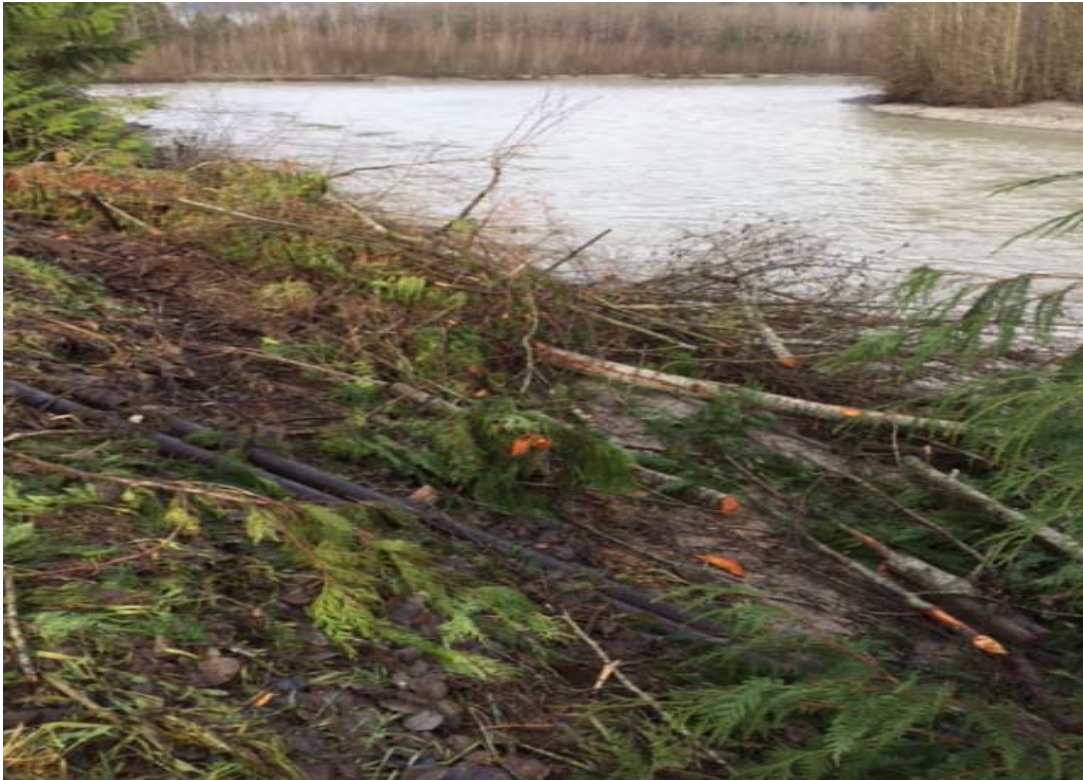
Dream Catcher Armor Damage – Nov 12 2016
