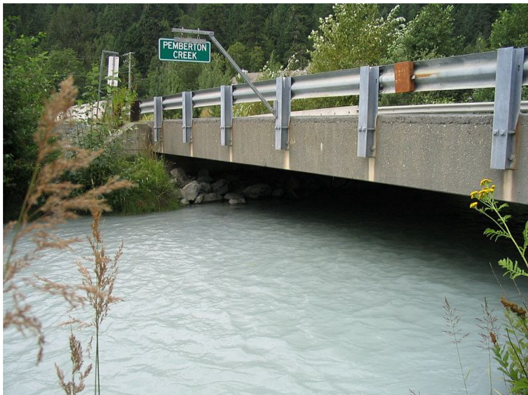
Photo 10 Downstream side of Hwy 99 bridge, Q = 2.4 \text{ m}^3/\text{s} (July 29, 2005).
