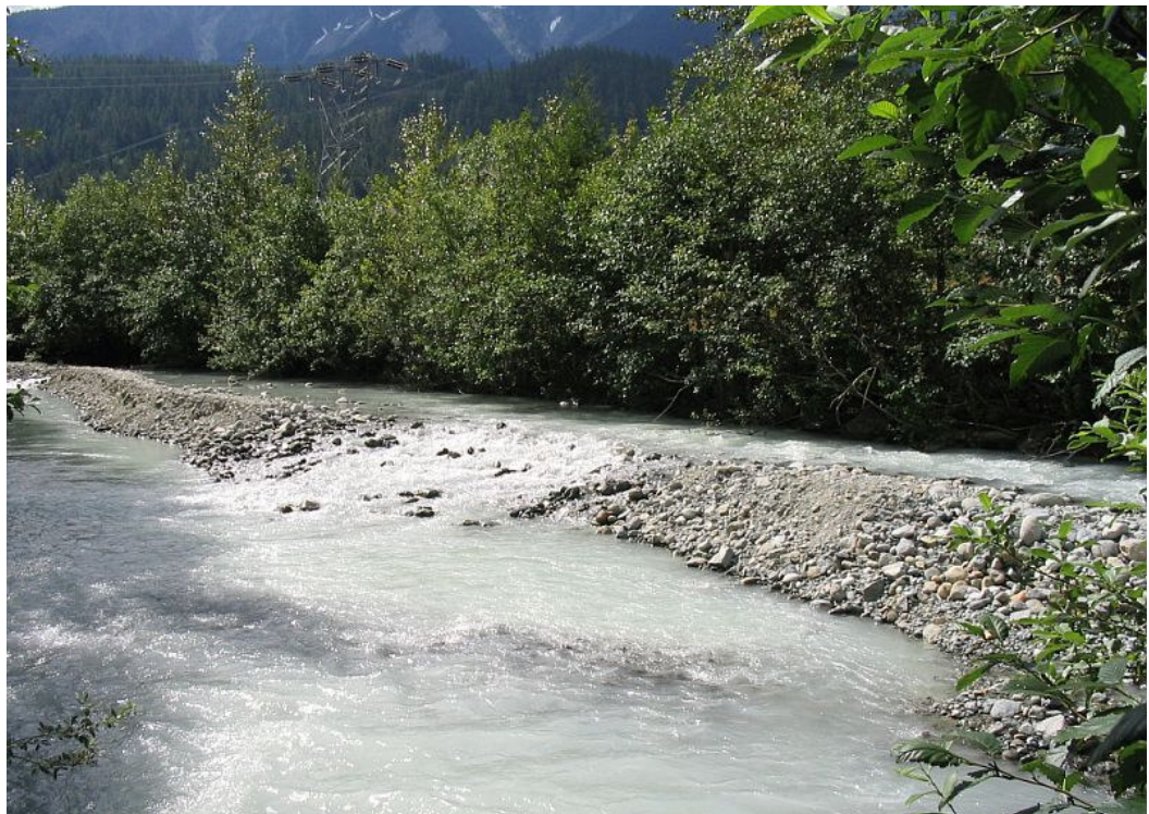
Photo 8 Looking downstream at large gravel deposit upstream of Hwy 99 bridge, post-removal (July 29, 2005).
