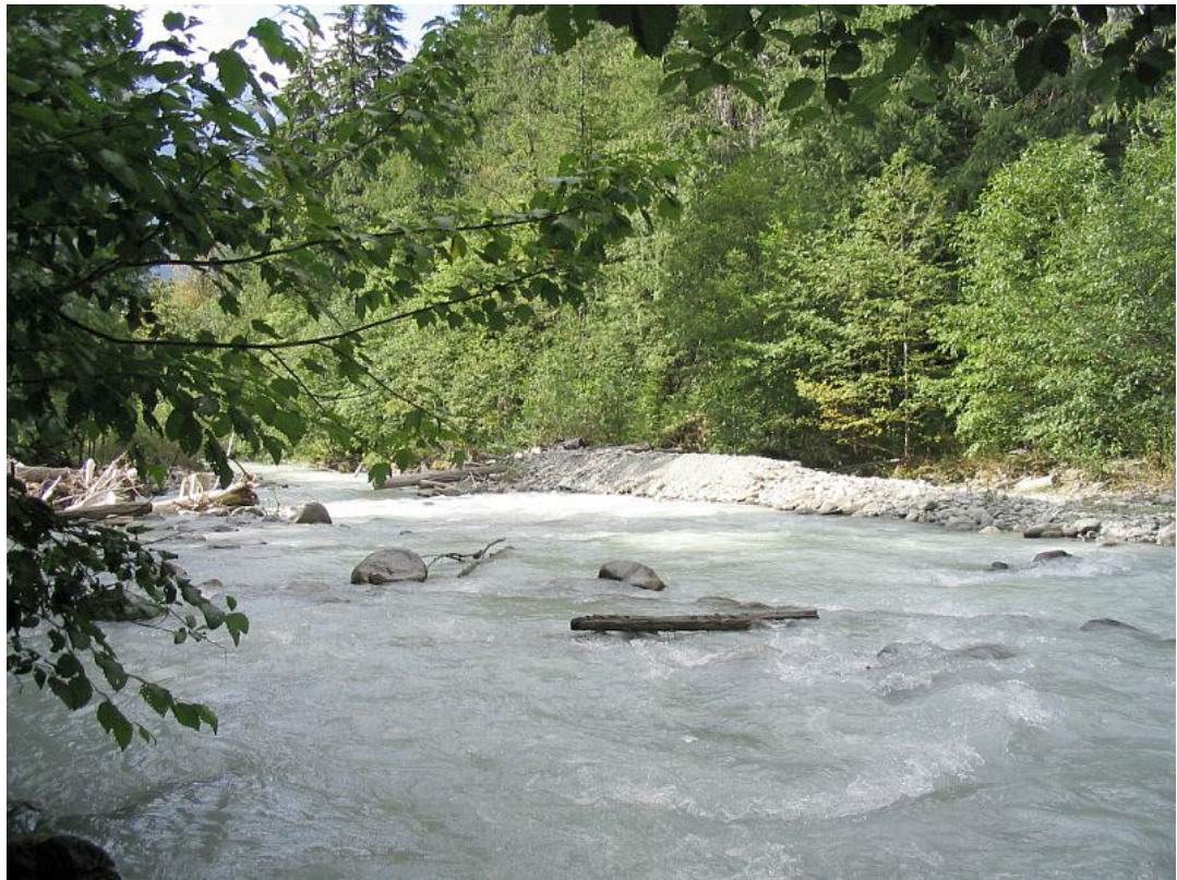
Photo 3 Pemberton Creek above BCR bridge, looking downstream. Note gravel bar on right bank.
