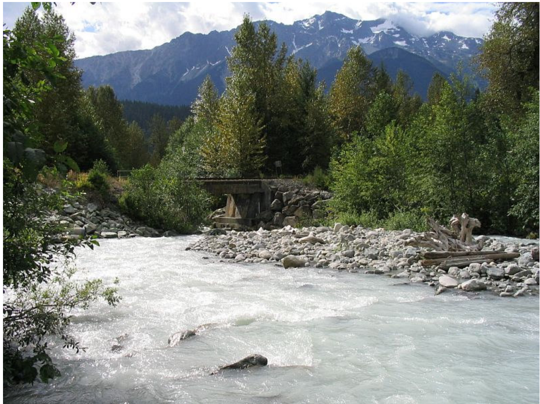
Photo 5 Pemberton Creek immediately upstream of BCR bridge (July 29, 2005).
