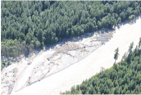
Photo E-7 Braided Reach Upstream of the Forestry Bridge (August 13, 2010) Shows New and Older Raked Material
