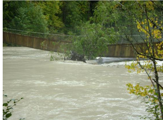
Photo 3-4 Footbridge (September 28, 2010) (Photo courtesy of Jeff Westlake)
