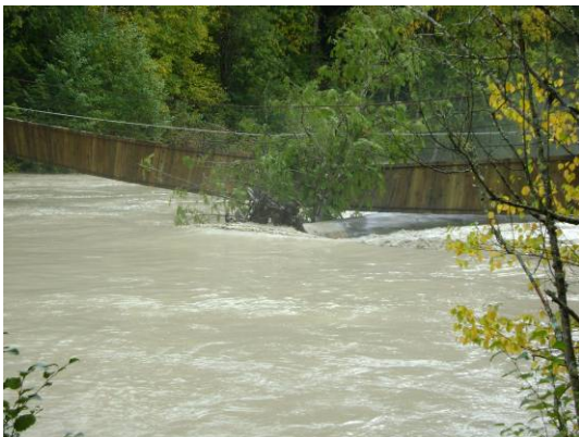
Photo 5-1 Footbridge Collecting LWD (September 28, 2010)
