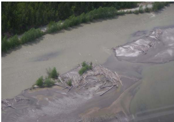
Photo F-9 Log Jam Upstream of Forestry Bridge Showing Evidence of Newer Racked Wood
